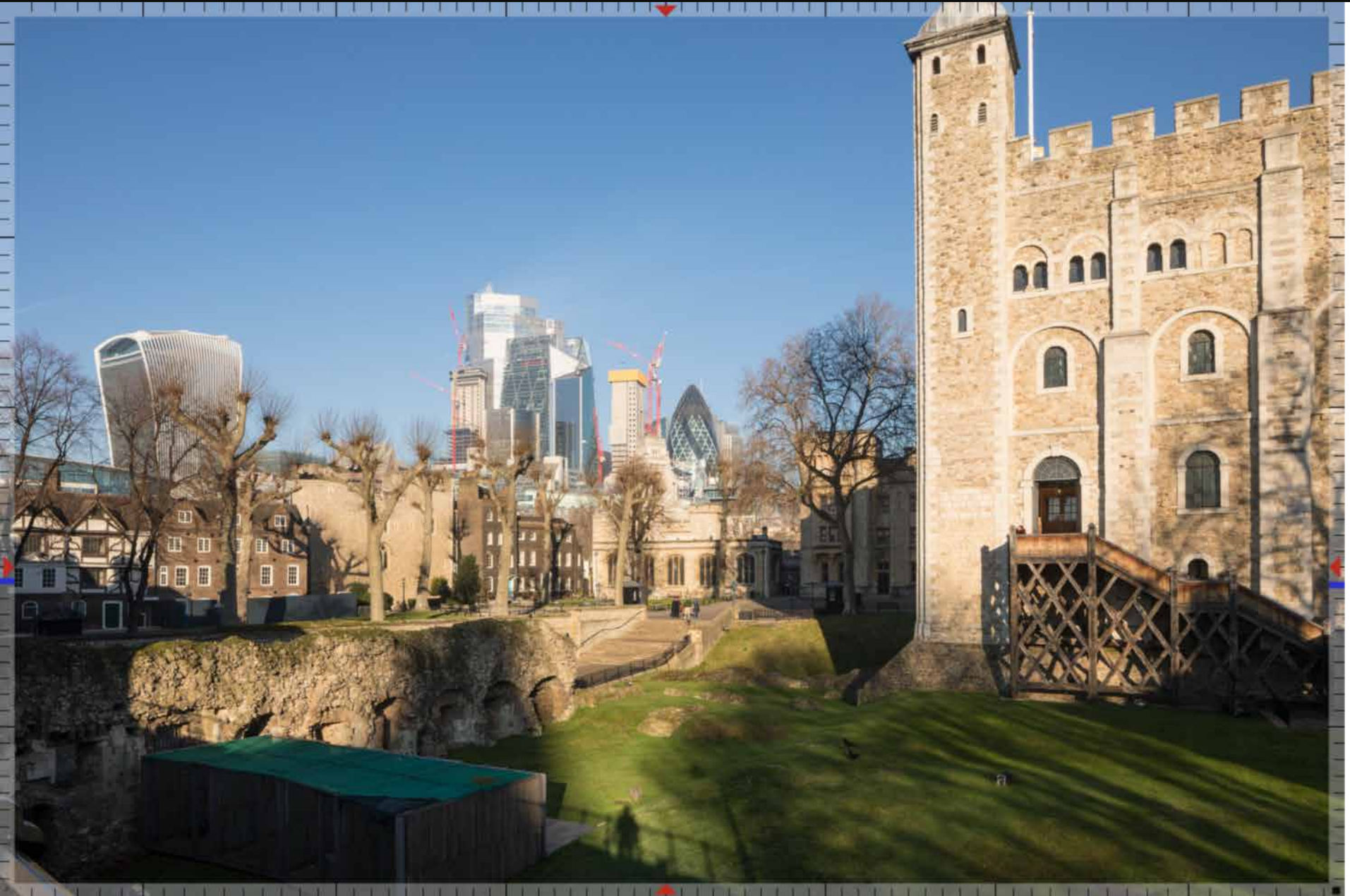
25 | Tower of London: Inner Curtain Wall - south
