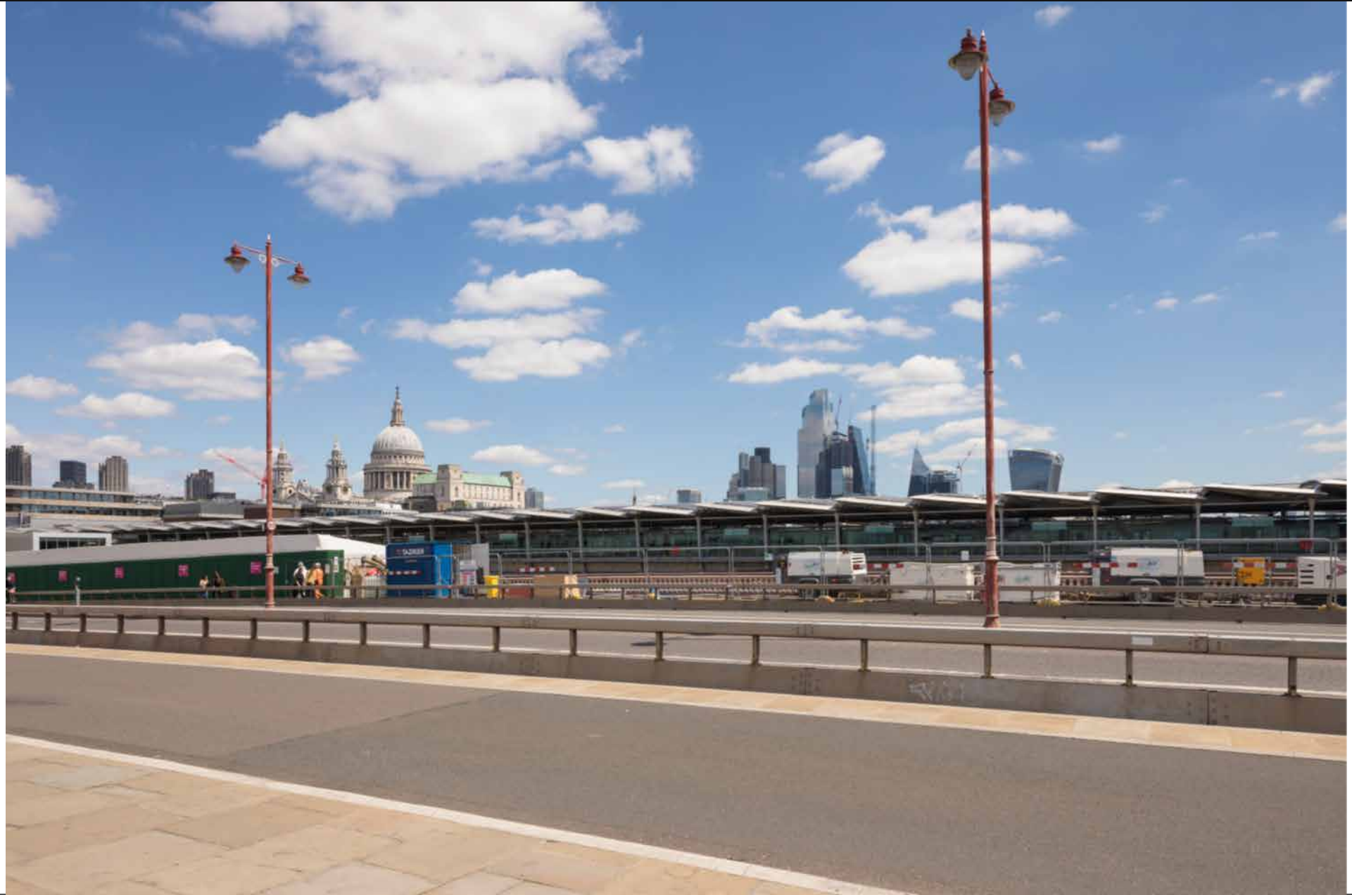
C07 | Blackfriars Bridge: LVMF 14A.1 position – centre of the bridge
