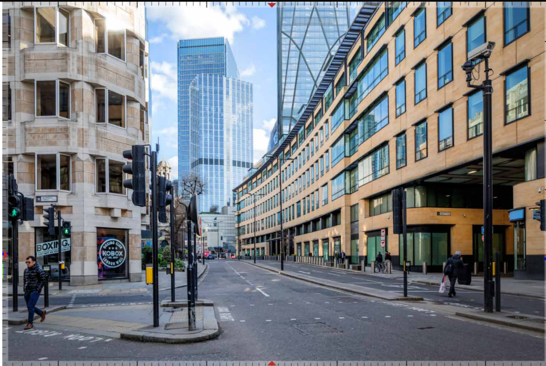
46 | London Wall, corner with Blomfield Street
