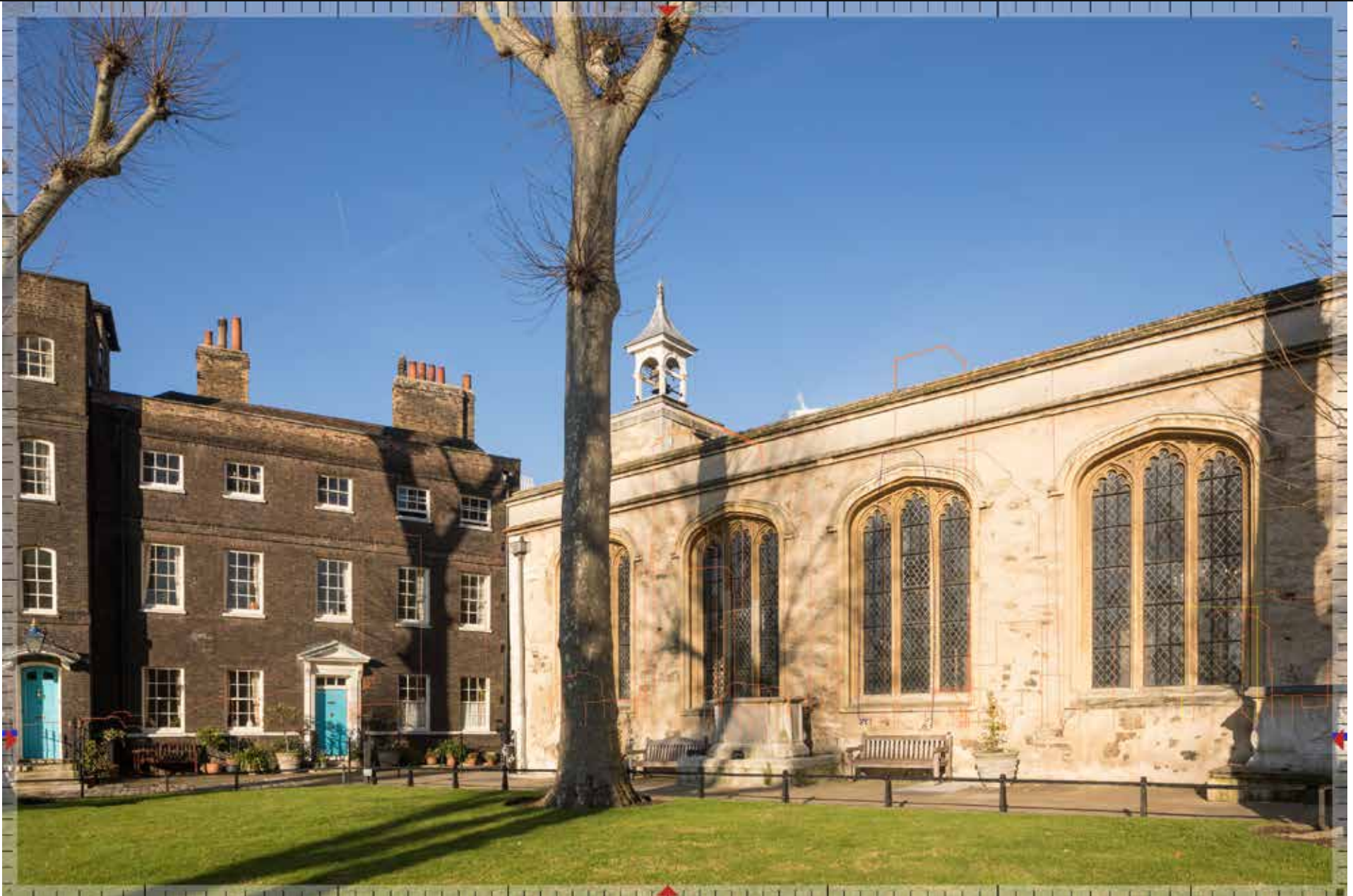
24 | Tower of London: the Inner Ward - Site of the Scaffold
