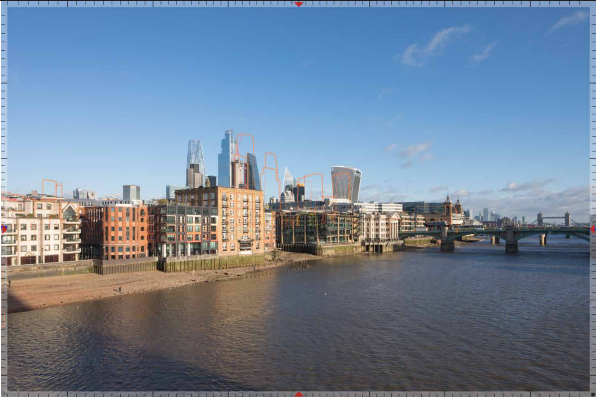
17 | Millennium Bridge - at the centre of the bridge
